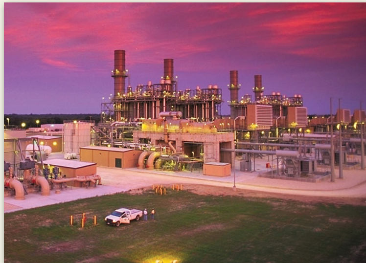
Calpine's Freestone Energy Center in Fairfield, Texas.
