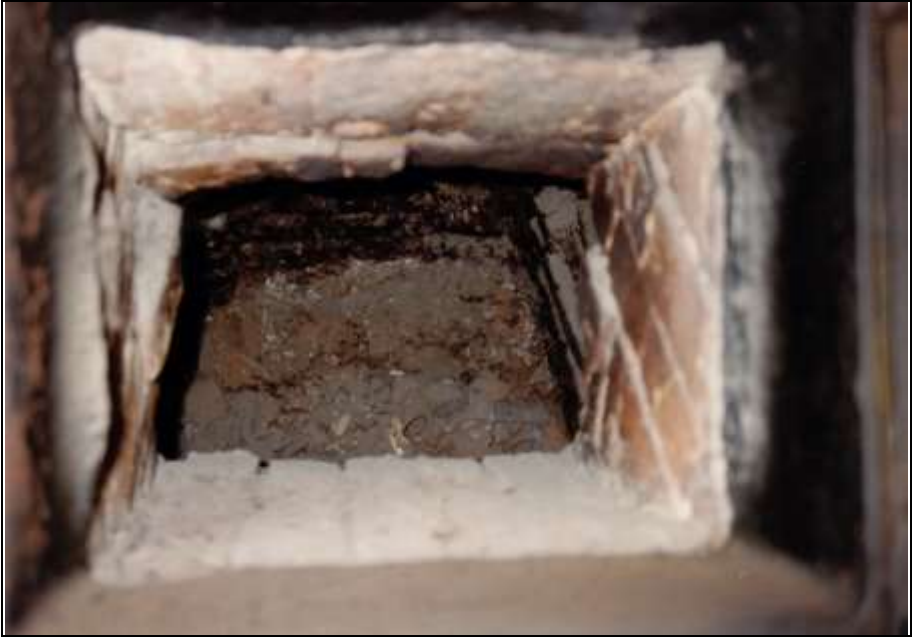
Photograph 163: as above, view through the coke-loading door into the gasifier.
