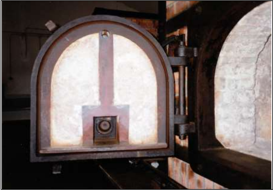
Photograph 129: TOPF coke-fired triple-muffle cremation furnace at Buchenwald Concentration Camp. Interior of the left-hand muffle door.
