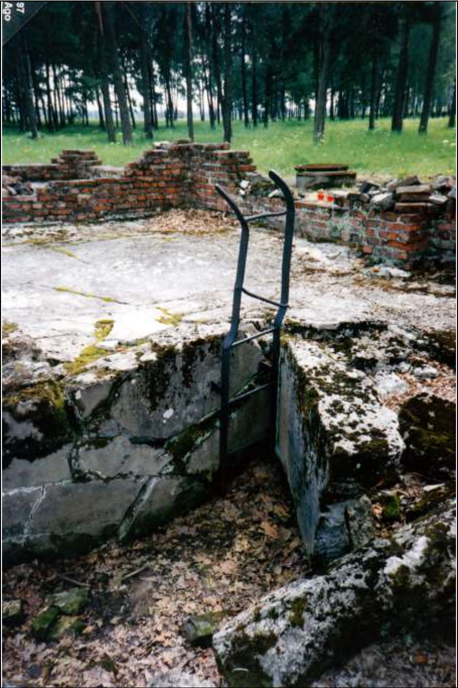
Photograph 232: as above. South service pit and access ladder.
