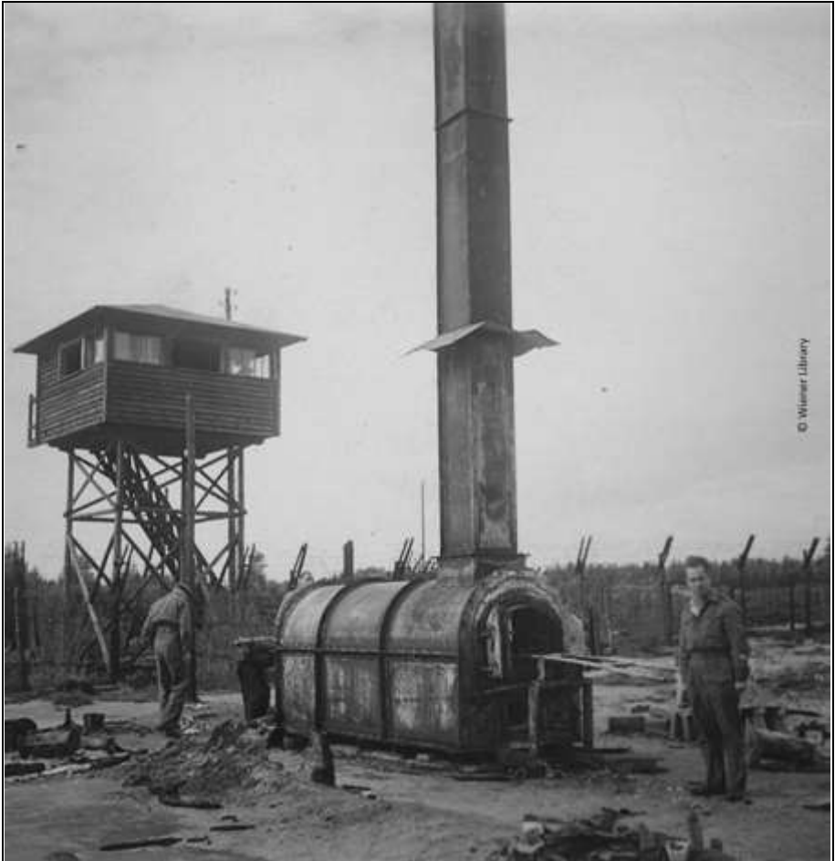
Photograph 339: KORI naphtha-fired cremation furnace at Bergen-Belsen Concentration Camp. Source: http://galleryhip.com/bergen-belsen-liberation.html , now removed.
