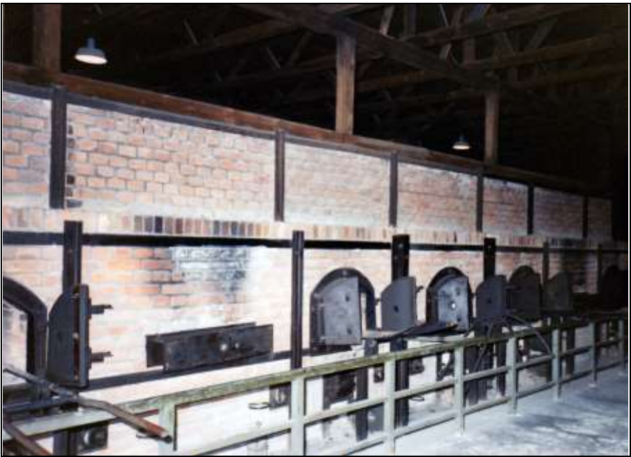
Photograph 287: Row of cremation furnaces with five muffles, front view.
