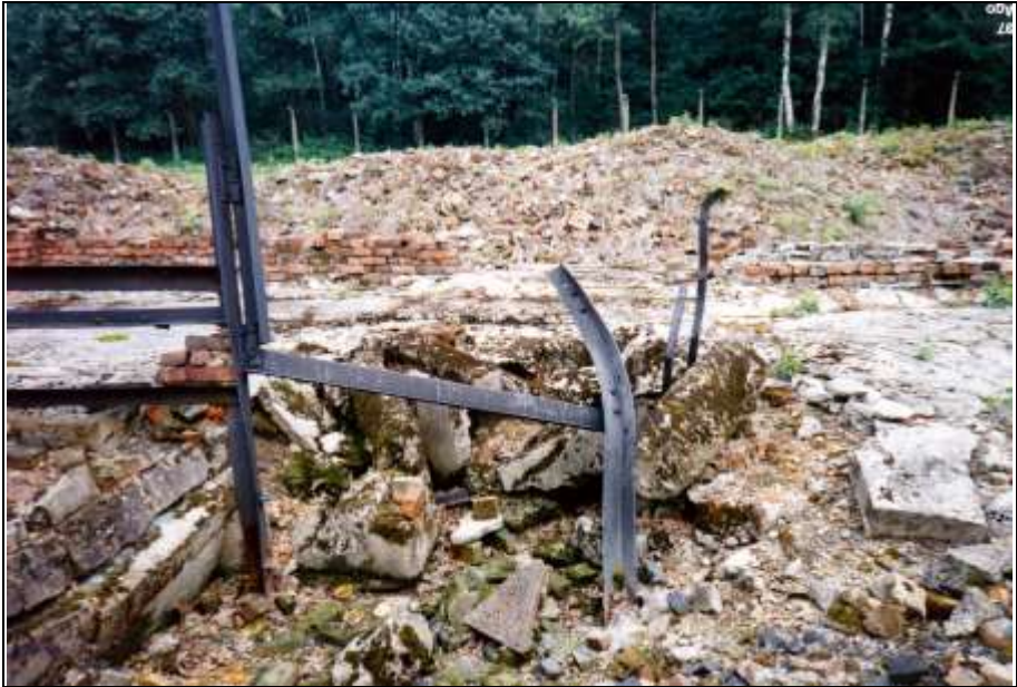
Photograph 230: as above; behind the iron frame: access ladder to the gasifier's service pit.
