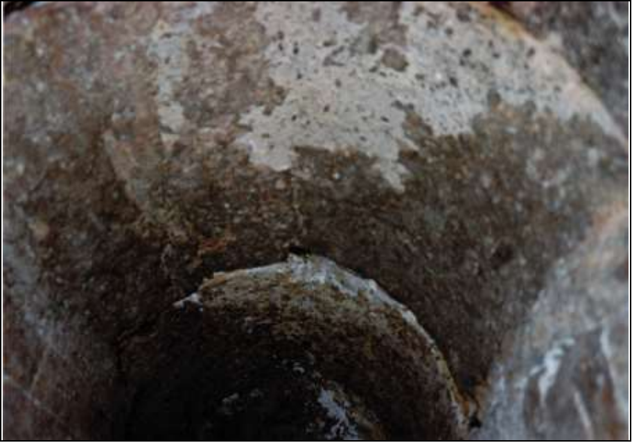
Photograph 26: Right-hand muffle: Vaulted muffle ceiling with the outlet of one of the pipes connected to a blower.
