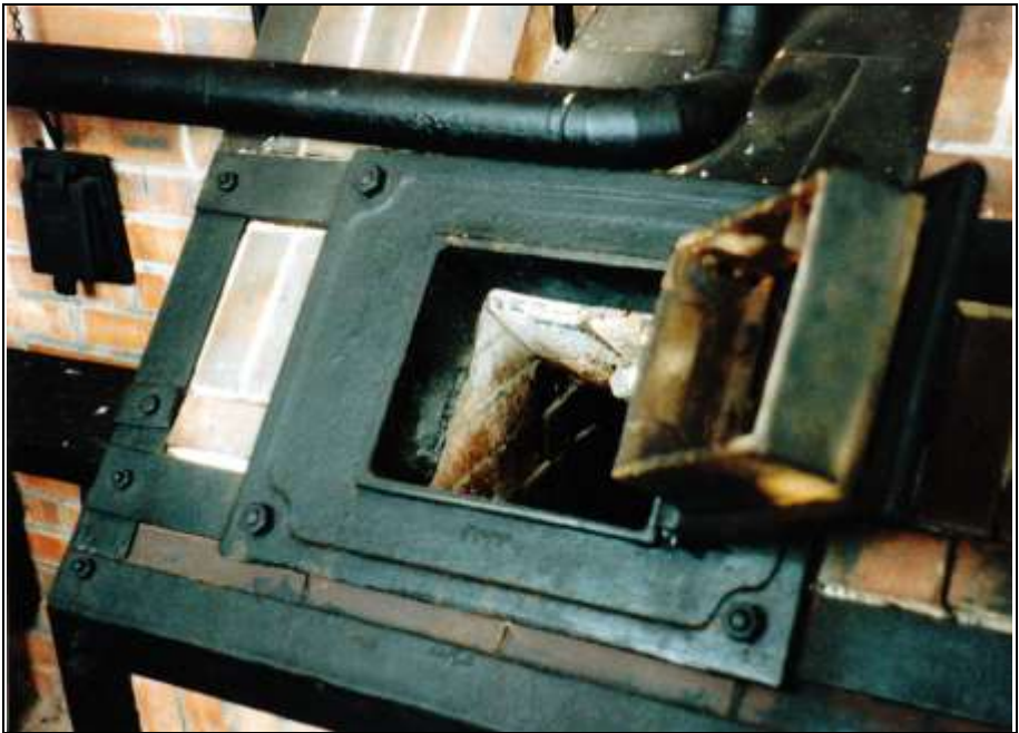
Photograph 162: as above, with opened coke-loading door.
