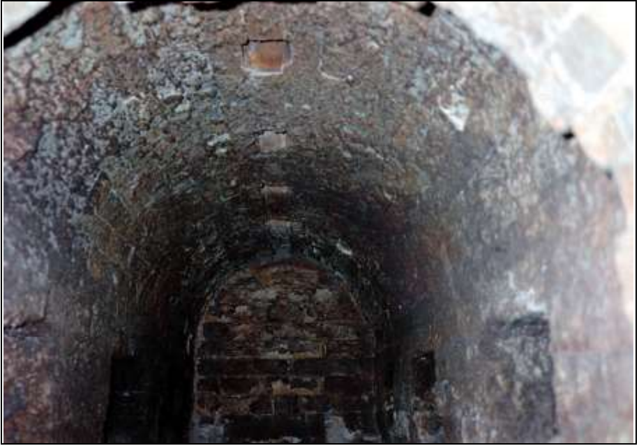
Photograph 137: as above, showing five of the rectangular inter-muffle openings, four square openings in the ceiling and one in the back wall for combustion-air supply.
