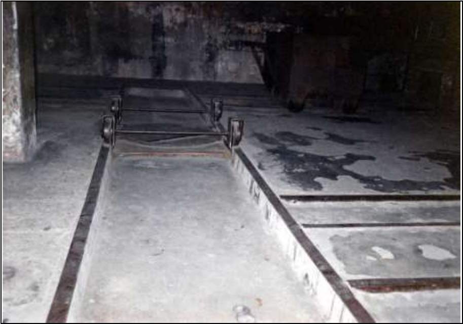
Photograph 105: Transverse rails and rotating platform (turntable).
