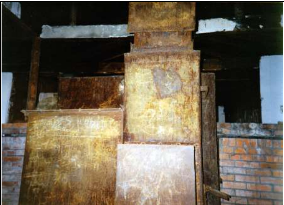
Photograph 48: Central part of the chimney.
