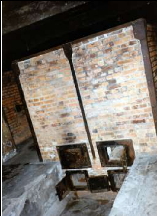
Photograph 97: Furnace No. 1, rear side. The furnaces were re-fabricated without gasifiers. The gasifiers' coke-loading doors are therefore necessarily in the wrong position over those of the ash-chamber doors. See Photo 78.
