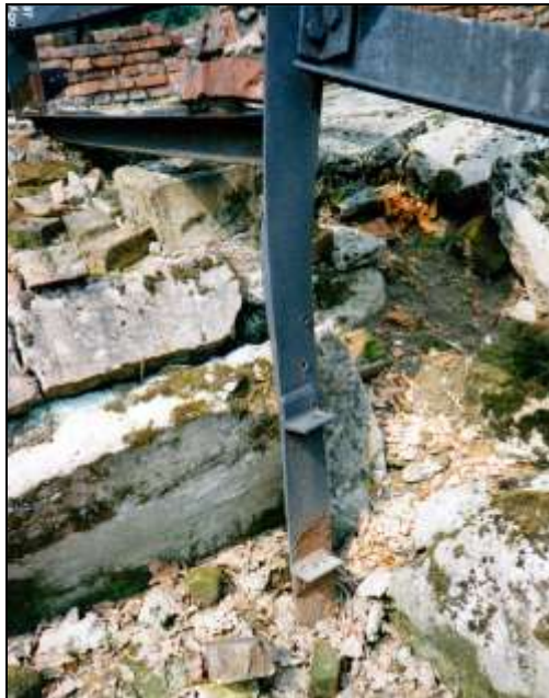
Photograph 231: as above. Detail of the north gasifier's frame irons (direction south-north). The two brackets visible below were used for mounting the gasifier's hearth door.
