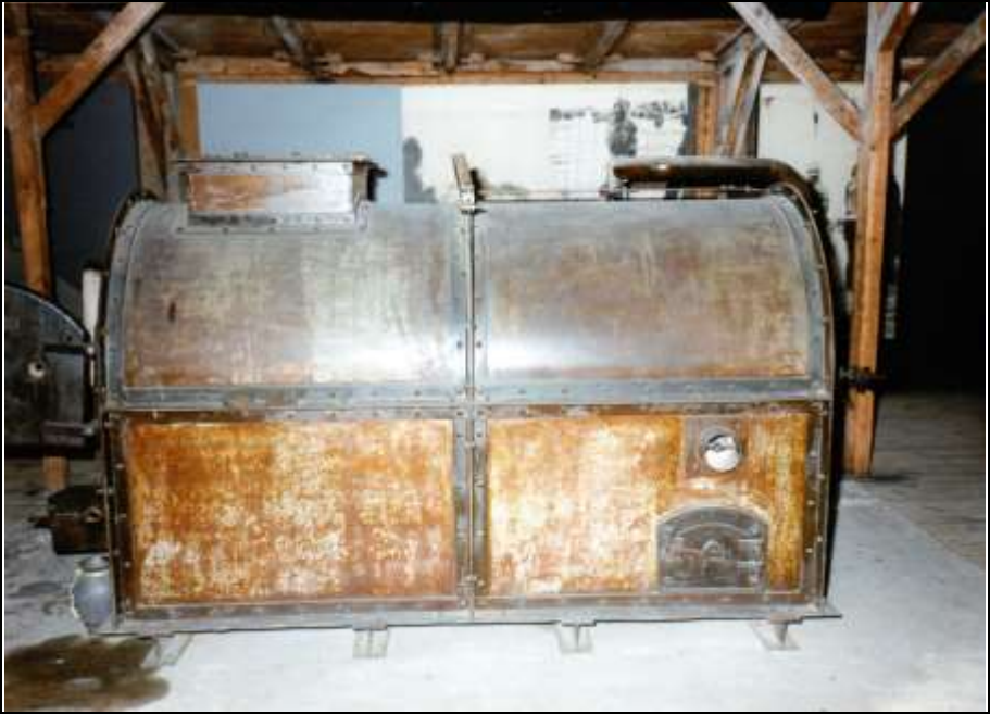
Photograph 326: right-hand side; bottom right: side inspection door beneath a combustion-air inlet.
