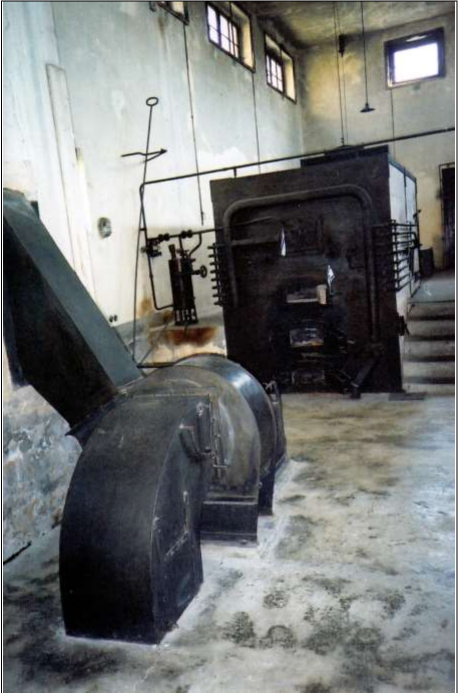
Photograph 357: as above, side view.
