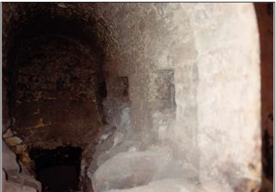
Photograph 142; as above, right-hand wall with rectangular openings to center muffle.
