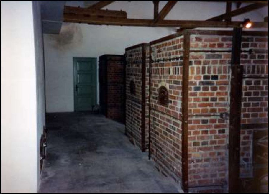
Photograph 258: Rear view of Furnaces Nos. 2 through 4 (front to back).
