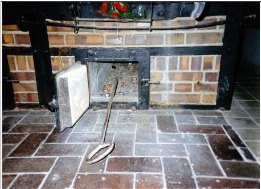
Photograph 71: Ash chamber of the right-hand muffle.
