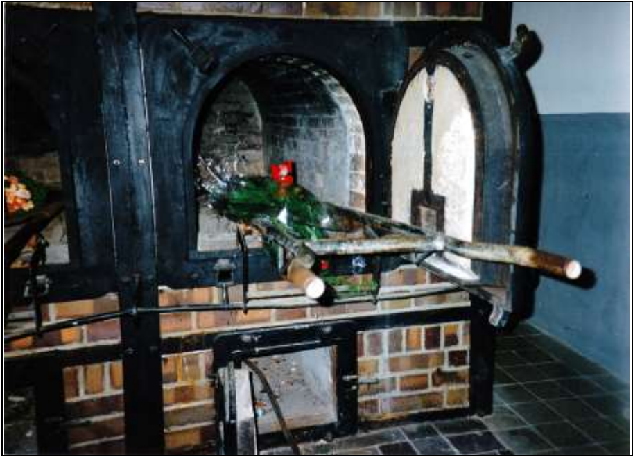
Photograph 70: Right-hand muffle with open ash door.
