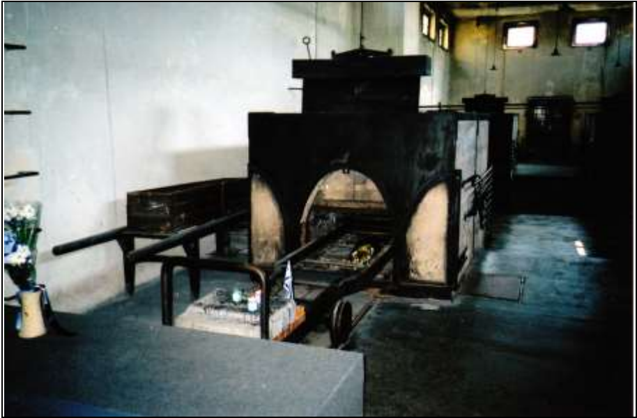
Photograph 346: Left-hand furnace of the front pair, front view, with the corpse-introduction cart.
