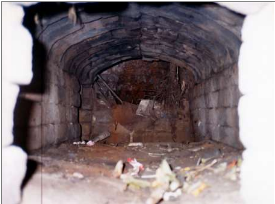
Photograph 273: The ash chamber of the left-hand muffle. Top: underside of the muffle's grate bars. On the left wall in the rear: opening connecting it with the auxiliary hearth. All the way at the back: the gasifier's pit.
