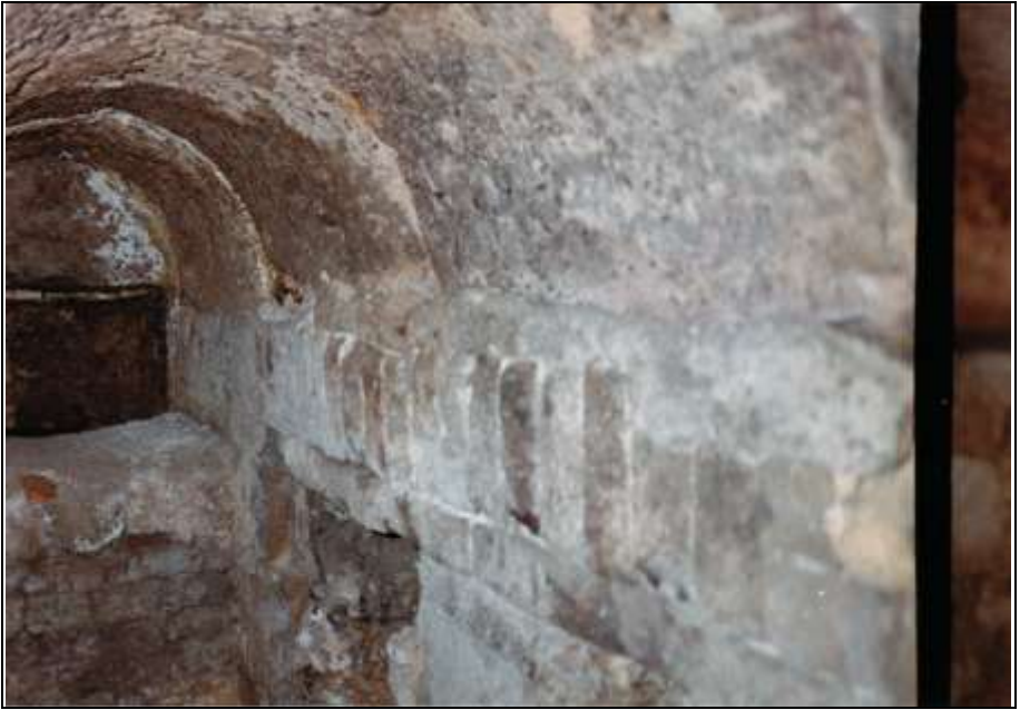
Photograph 28: Right-hand muffle: lateral wall of muffle and ash compartment with an opening connecting it to the gasifier.
