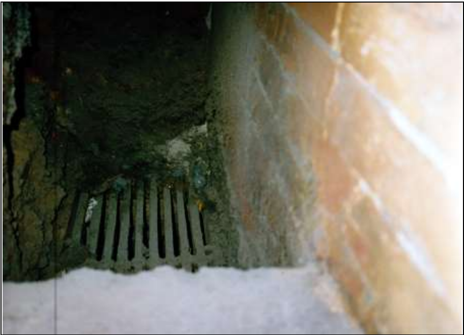
Photograph 263: View into the main gasifiers.
