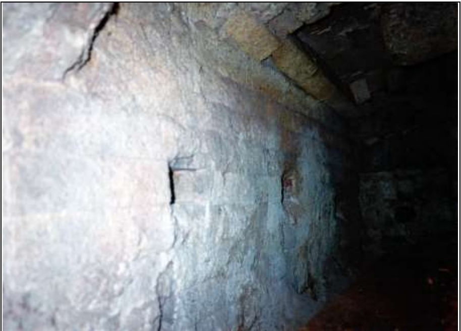
Photograph 241; as above, close-up of combustion-air-supply holes.
