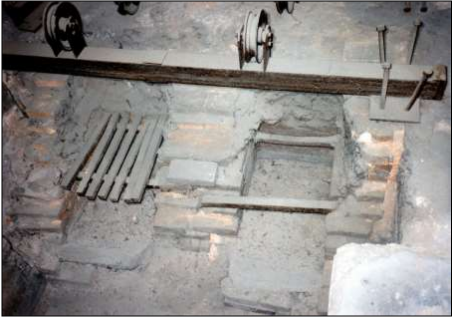
Photograph 101: as above, seen from the rear: original grate of the left-hand gasifier and the two transverse support bars of the right-hand grate. The bar with the rollers, originally attached to the ceiling, was used to operate the furnace's two flue dampers.
