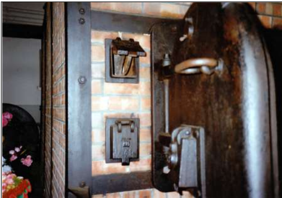
Photograph 153: as above, both doors of the combustion-air channels.
