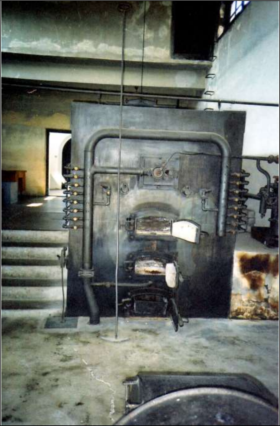
Photograph 348: as above, rear view.
