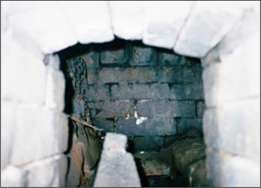
Photograph 281: as above. View into the auxiliary gasifier. Background: the wall of the muffle's ash chamber. Foreground: the end of an iron bar from the auxiliary hearth grate.
