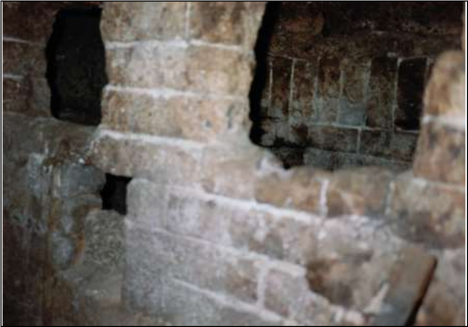
Photograph 20: Left-hand muffle: partition wall with inter-muffle openings.
