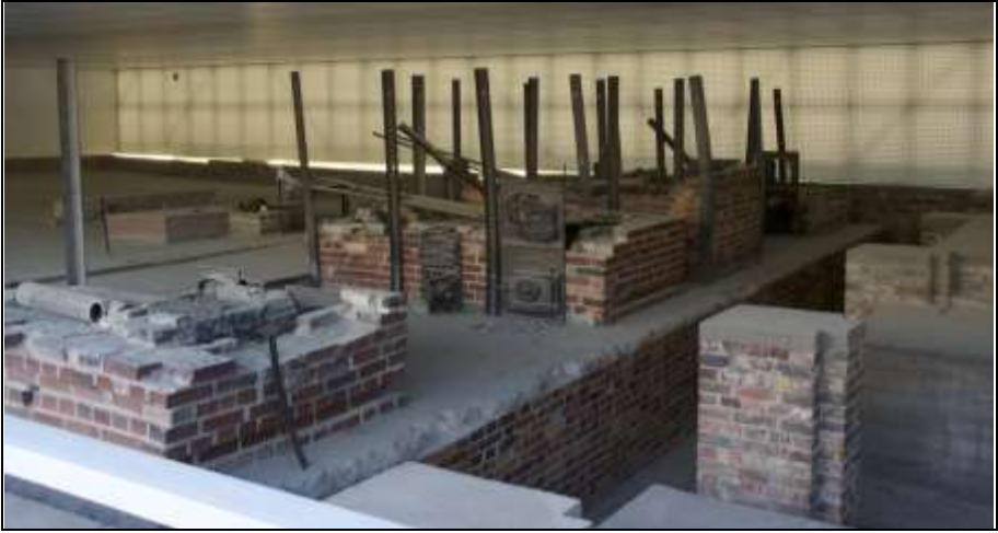
Photograph 337: Ruins of the KORI coke-fired cremation furnace at Sachsenhausen Concentration Camp. Source: http://snapeatrepeat.com/tag/sachsenhausen-concentration-camp/ , now removed.
