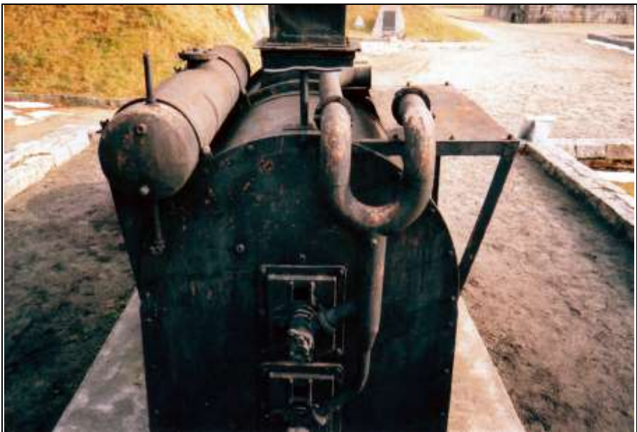
Photograph 333b: as above. The air pipes were originally connected to a blower installed on the shelf to the right.
