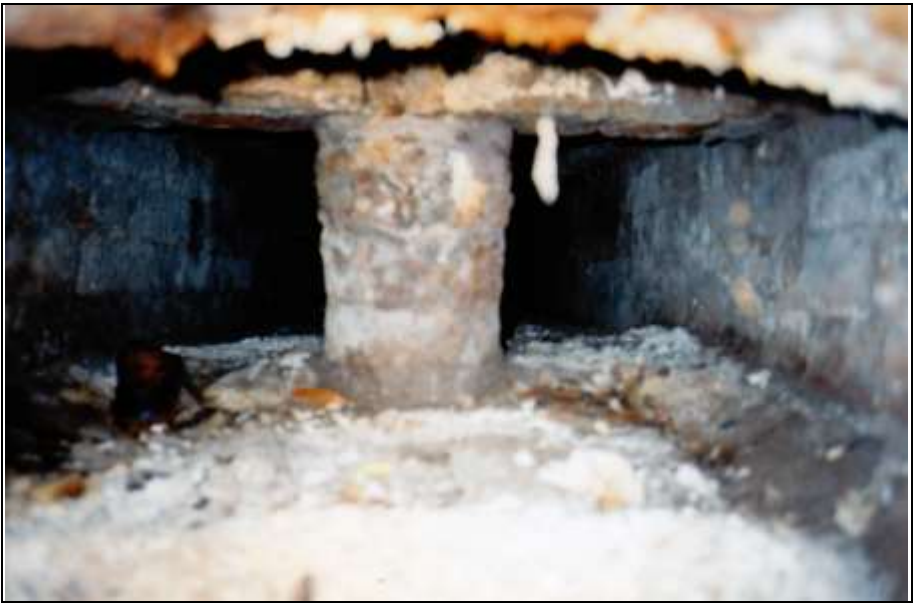
Photograph 354a: as above; close-up.
