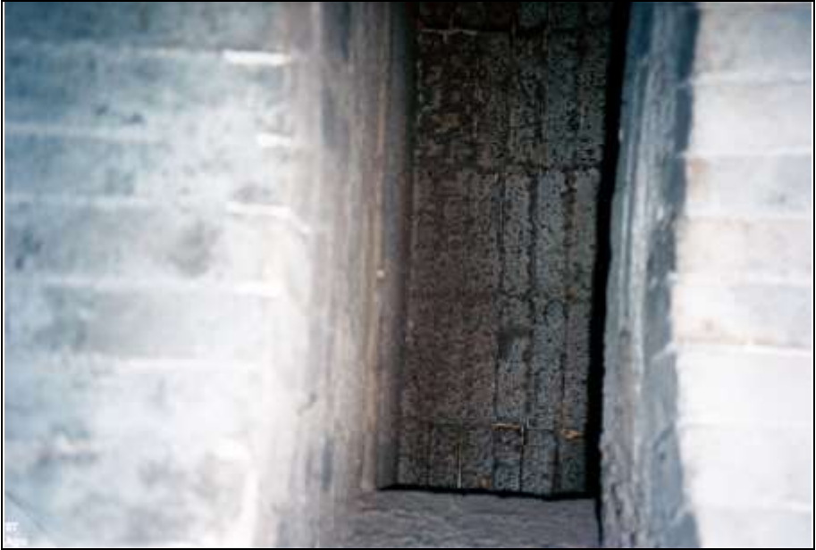
Photograph 302: Vertical duct of the flue-gas outlet.
