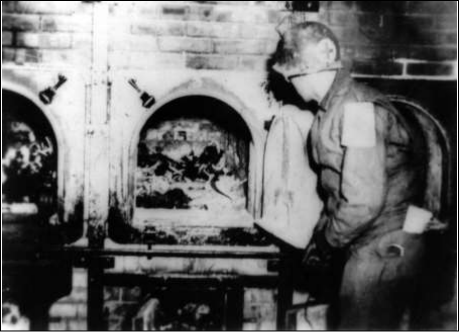
Photograph 206: A U.S. soldier in front of the central muffle of the TOPF coke- or naphtha-fired triple-muffle cremation furnace at Buchenwald Camp. U.S. Army photo of 1945.
