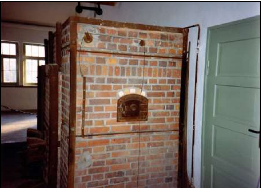
Photograph 259: Rear view of the first furnace; inspection door of the vertical smoke duct. Wire cable and pulleys for operating the smoke-duct damper, visible in Photo 258 on the floor at the bottom of the furnace.
