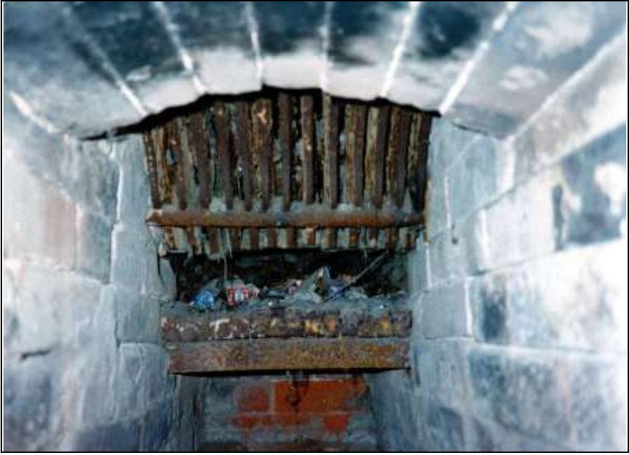
Photograph 246: gasifier grate.
