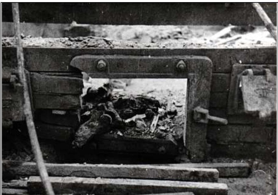
Photograph 227: as above, ash chamber's door frame of the muffle located in the north-western corner. Visible on the right is the door of the ash chamber's combustion-air channel.
