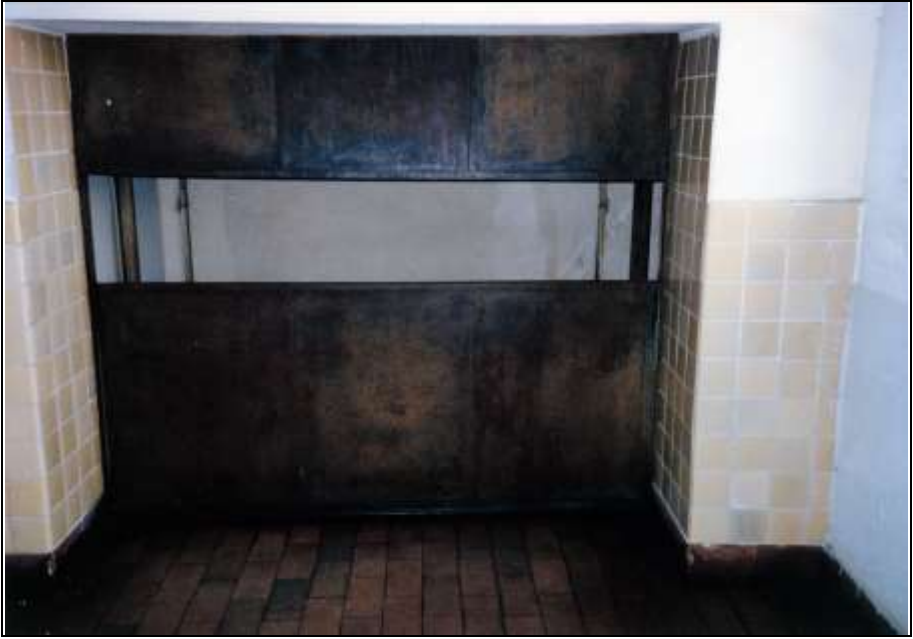
Photograph 214: as above, elevator door in the cremation hall, ground floor.
