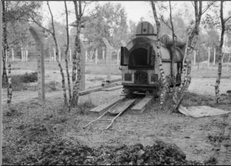
Photograph 344: KORI naphtha-fired cremation furnace at Vught Concentration Camp. Source: http://ww2today.com/wp-content/uploads/2014/11/vught-crematoria.jpg .
