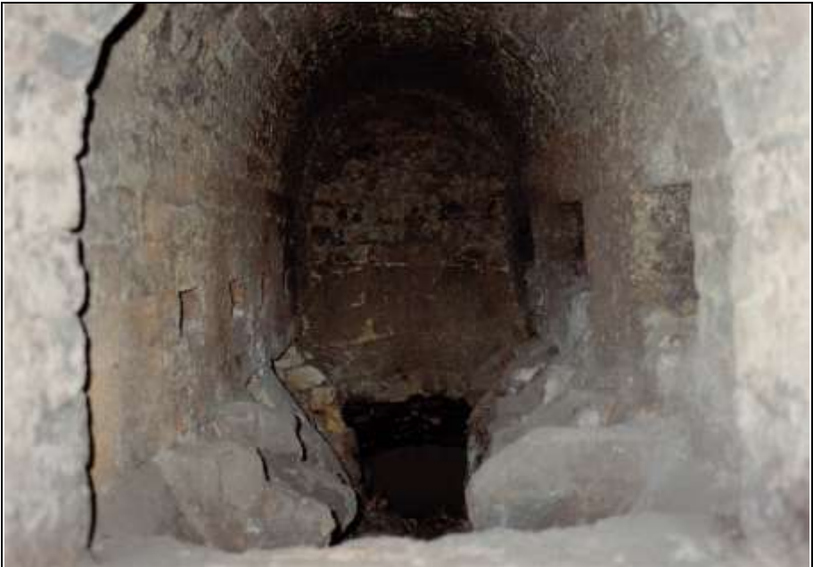
Photograph 140: Coke-fired triple-muffle furnace, left-hand muffle. Left wall: square openings of the combustion-air feed. Bottom: wall sloping into the ash chamber). Center bottom: opening to the gasifier. Right-hand wall: rectangular inter-muffle openings. The muffle-grate bars have been ripped out.
