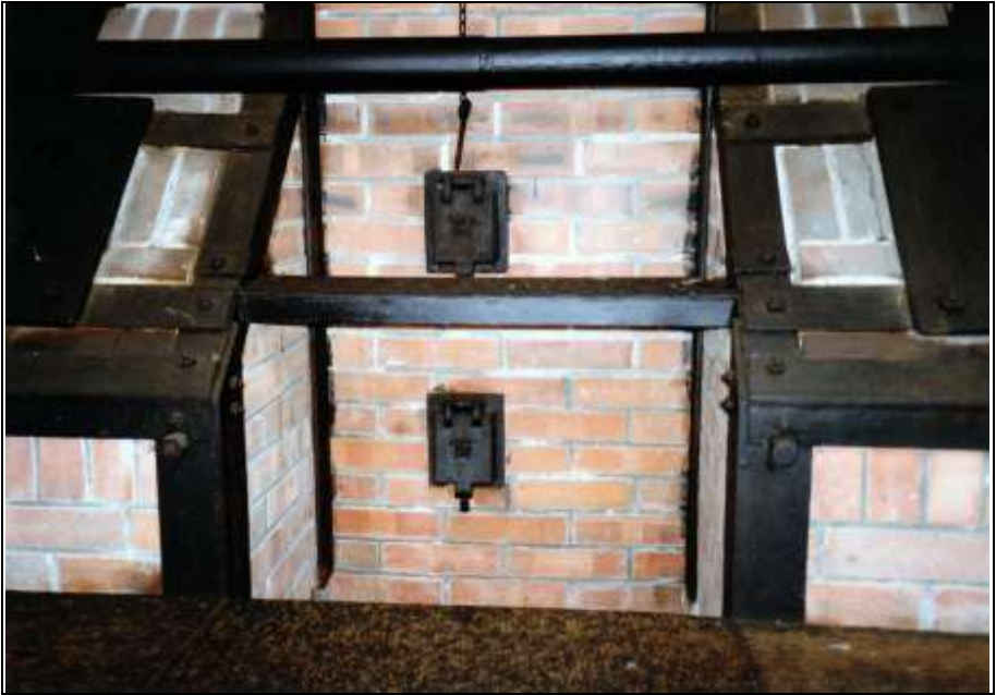
Photograph 169: as above; doors to the muffle's (top) and the ash chamber's combustion-air channel (bottom).
