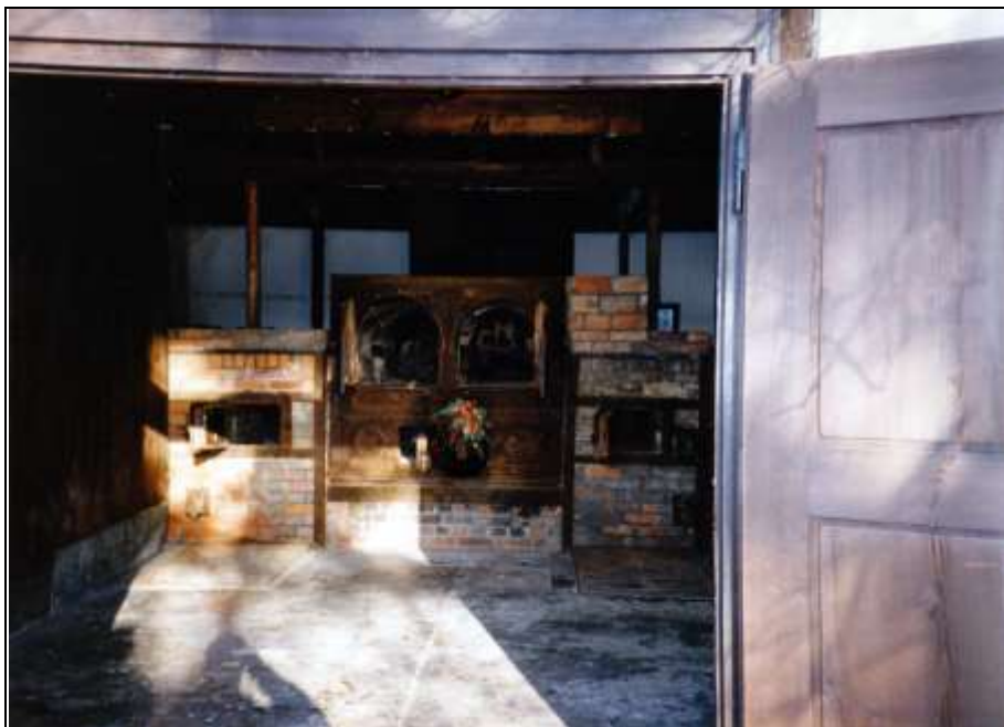
Photograph 36 (top) and 36a (bottom): Original furnace body of coated sheet metal with masonry gasifiers added to its sides.
