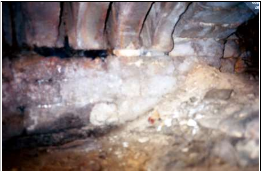
Photograph 284: as above; right-hand wall of the muffle's ash chamber as seen from the auxiliary gasifier's ash chamber; top: vaulted muffle-grate bars.
