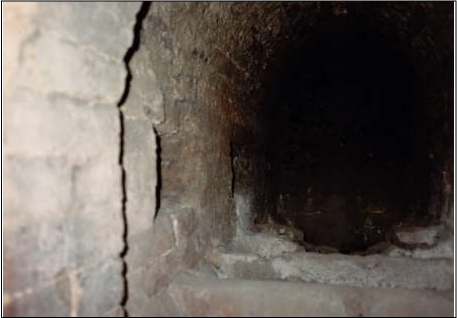
Photograph 145: as above, right-hand muffle, left-hand wall with rectangular openings to the center muffle.
