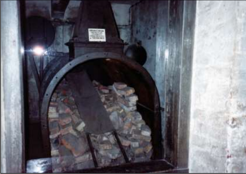
Photograph 330: Front view of the furnace. The interior of the furnace was completely destroyed. At the top the conical chimney (center), the blower (left) and the naphtha tank (right).
