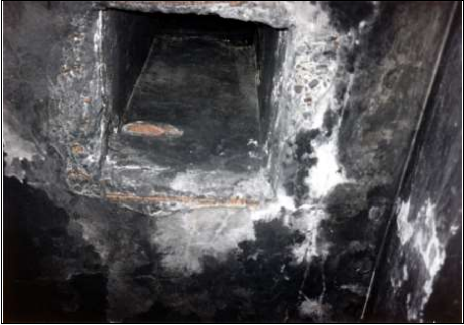
Photograph 103: Ceiling of the furnace hall: ventilation opening over Furnace No. 1.
