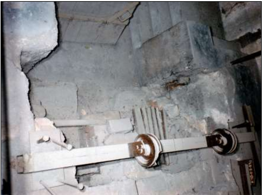
Photograph 100: Ruins of the foundations of Furnace No. 3: service pit and the gasifier hearths seen from the top.
