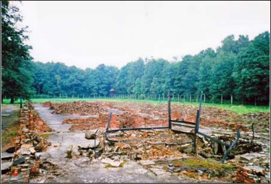
Photograph 228: Ruins of Crematorium V (1997). Wrought-iron frame of the Topf eight-muffle furnace (direction west-east).
