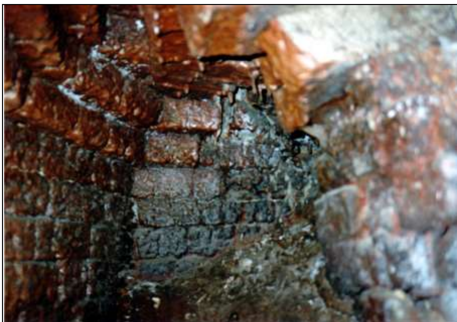
Photograph 5: Left-hand gasifier: Inside view, with the first opening connecting it to the left-hand muffle. The refractory brickwork shows evidence of fusion. (For two similar images, see Photographs 315f., which were placed later out of order.)
