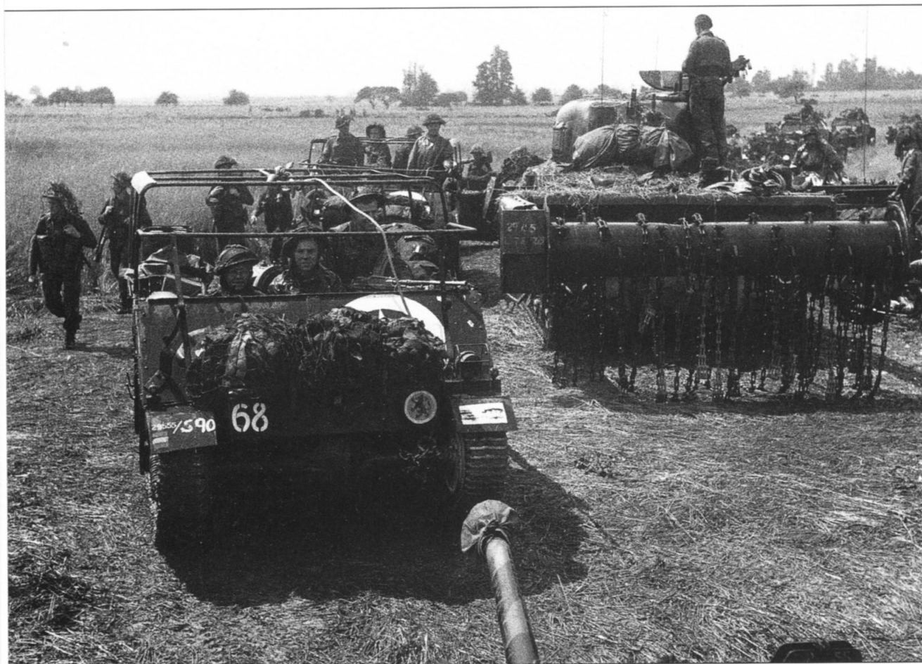
■ Above: Flail tanks of the British 79th Armoured Divisions were used to clear paths through German minefields.
