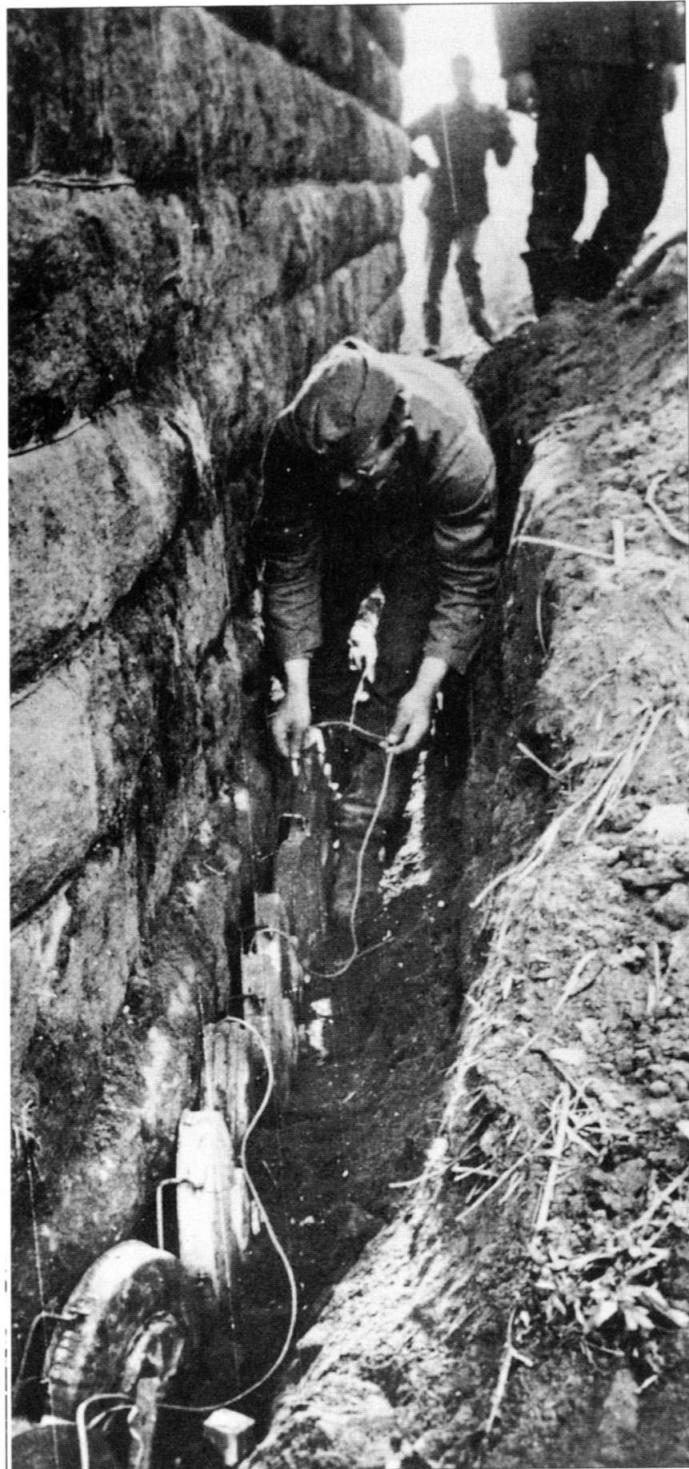
LEFT: German engineers rig a series of Teller-Mines, including what appear to be TMI 35 and 35 Stahl, to destroy a building during a retreat west in Russia.
