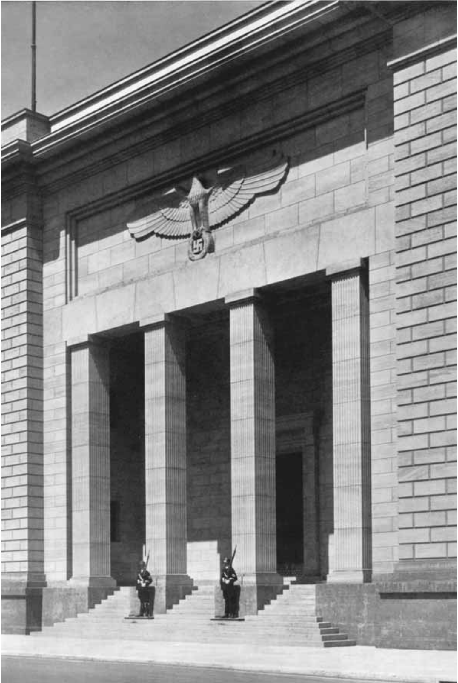
WESTPORTAL AN DER VOSS-STRASSE
