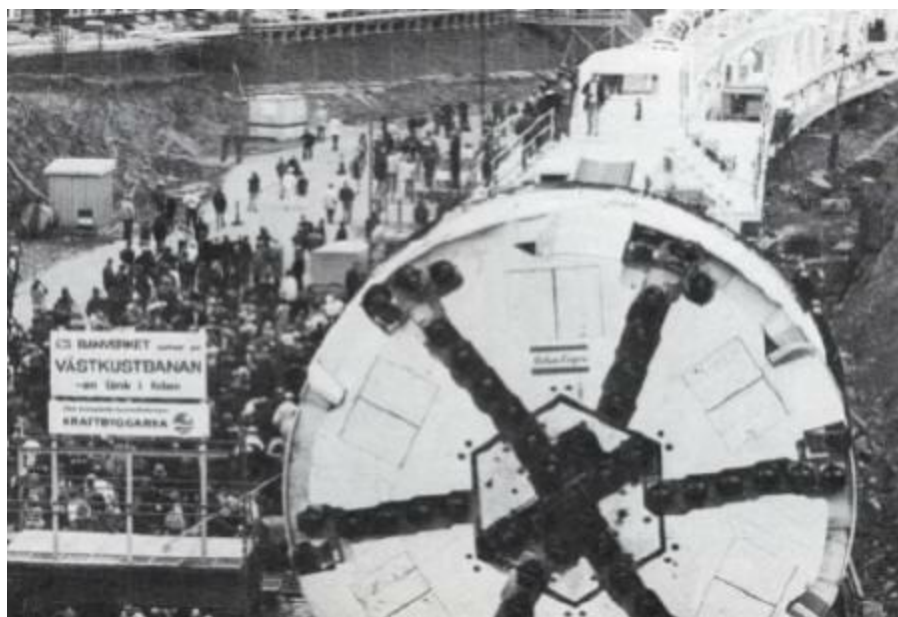
A Large, Conventional German Tunnel Boring Machine 57
