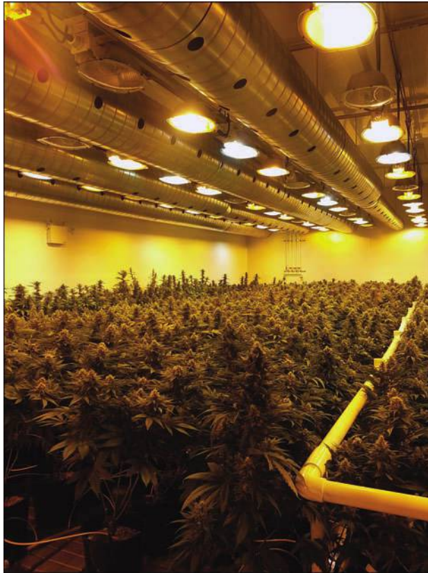
FIGURE 14.4 Medical marijuana growth facility of Tweed Inc. (Smith Falls, Ontario, Canada). The light installation shown here features alternating high-pressure sodium and metal halide lamps in rows between ventilation pipes to regulate temperature. Photo courtesy of Steve Naraine.
