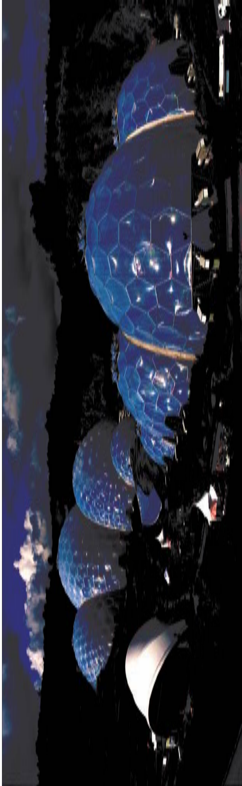
FIGURE 14.9 The geodesic domes at the Eden Project in England. Photo courtesy of Jürgen Matern (CC BY SA 2.5).
