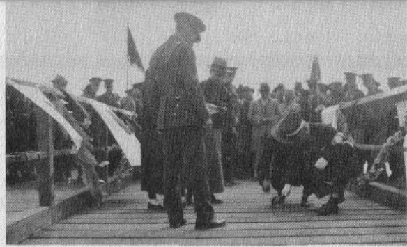
Driving the last four spikes into "Butler Bridge," built by the Marines at Peichang, in October, 1928, to replace a bridge on the Tientsin-Peking road washed out by storms
