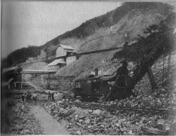
Building the Panama Canal, 1910
