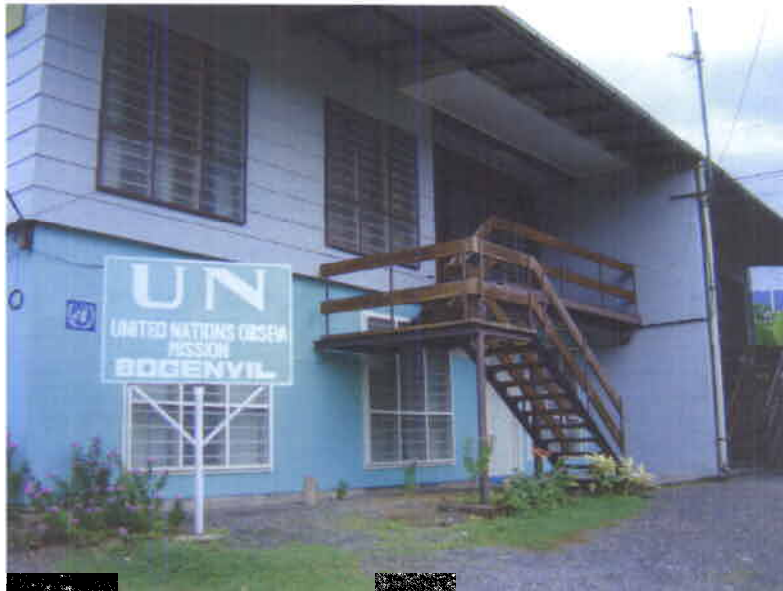
Photo 1 - UNOMB Office Premises at Arawa, Bougainville
