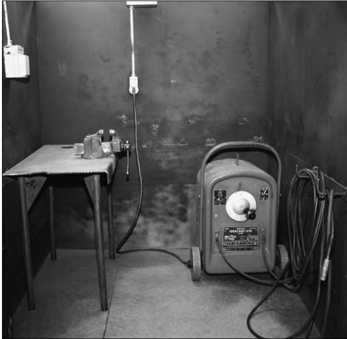
Figure 4-1: A well-equipped welding area setup, this one for stick welding.
