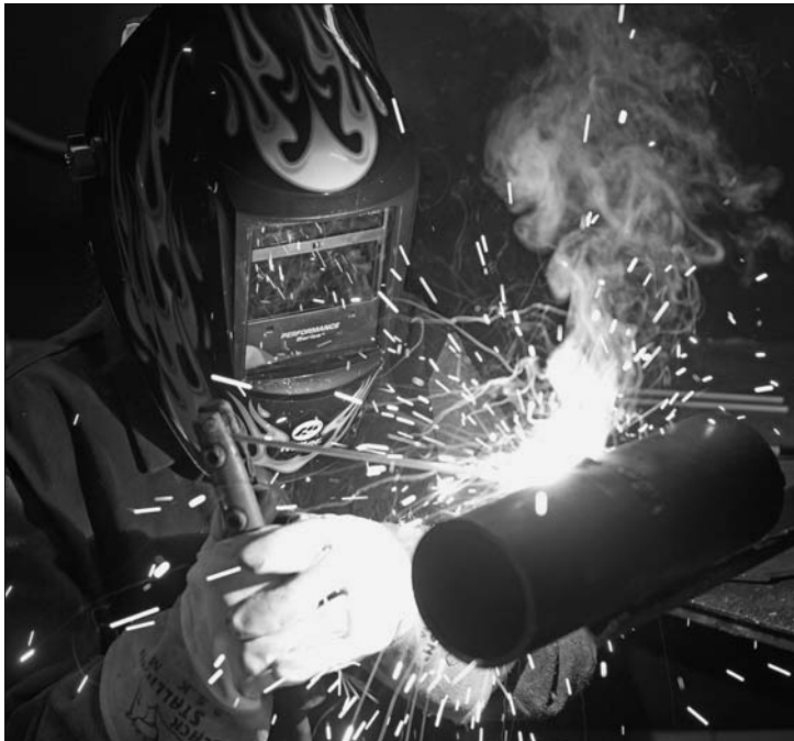
Figure 14-1: Steel pipe being stick welded.
