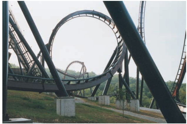
Welded joints are a critical component of structures
