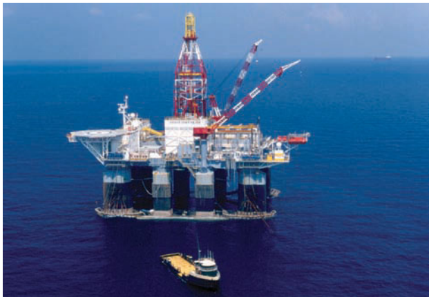
Figure 4.1 Large welded oil platform
