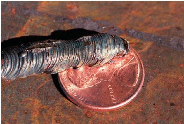
Figure 2.37 Weld separated from the plate There is no fusion between the weld and plate.
