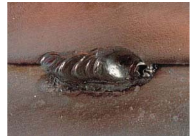
Figure 2.39 The tack weld should be small and uniform to minimize its effect on the final weld Courtesy of Larry Jeffus
