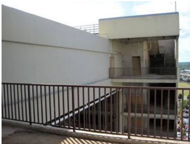
The balcony below, looking over to the opposite side
