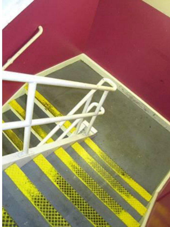
Looking down the stairway from the entry room
