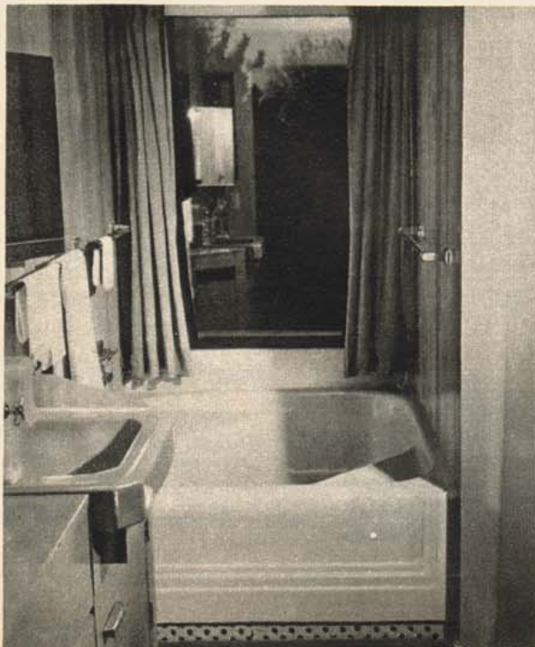
Heated air enters the bathroom through a duct beneath the tub, warming the bathtub and the floor
