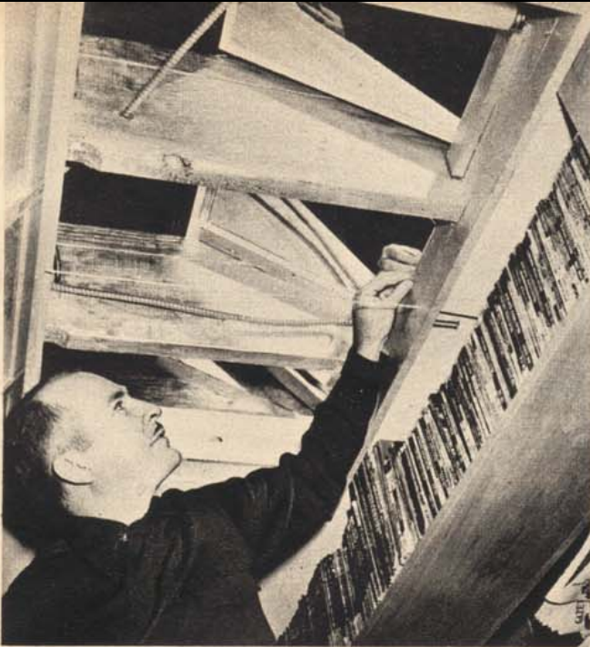
Skylight panels have mirrors which reflect sunlight into house. Behind panels are tubes for night lighting
