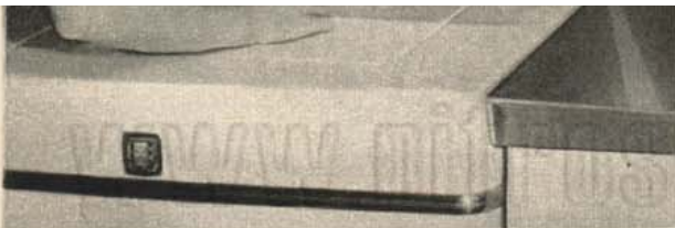
Trash goes through a hinged partition in kitchen wall, falls into a storage bin outside the house
