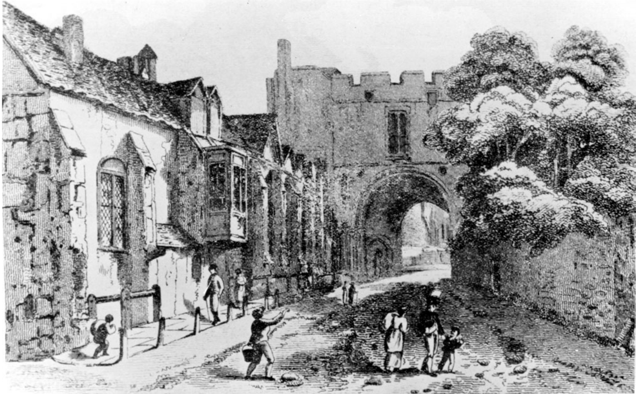
5 The old King's School in the Almonry buildings at Canterbury, viewed from the south
