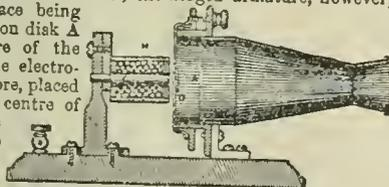
FIG. 3.—Bell's second telephone; one-fifth full size.
