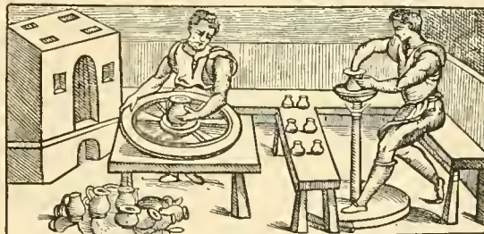
FIG. 55.—Two forms of Italian potter's wheels, about 1540.
