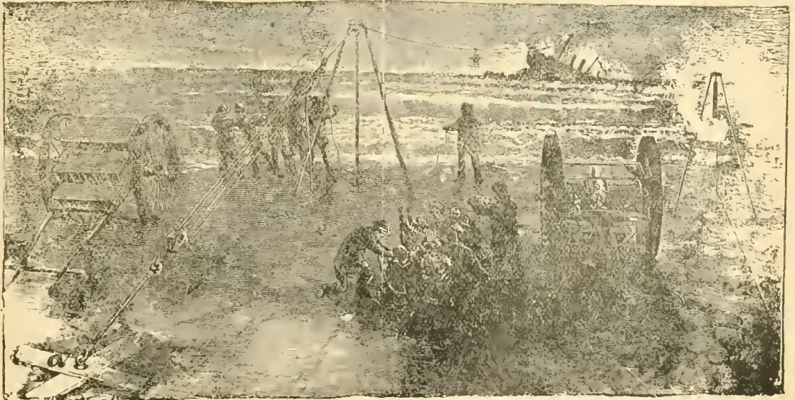
Fig. 11—NIGHT WRECKING OPERATIONS ILLUMINATED BY "SAUSAGE-LIGHT."
