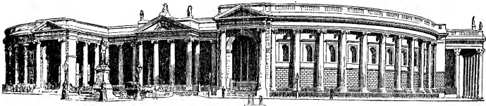
FIG. 85.—Bank of Ireland, Dublin.
