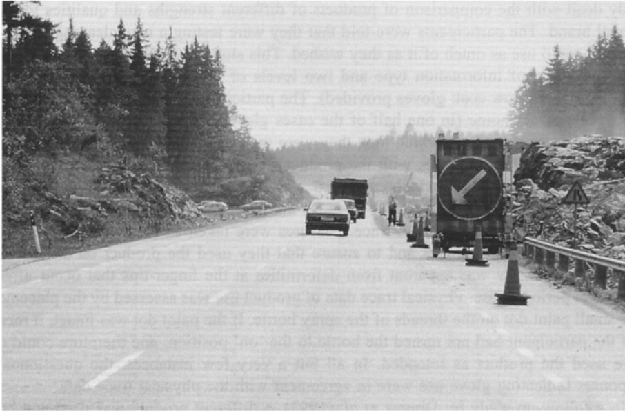
Figure 4.3 Swedish truckers were sent a cassette audio tape that included safety information about hazardous driving at work zone areas. Compliance was assessed by measuring the truck speed and distance of the vehicle to the side of the work zone (from Summala and Pihlman, 1993).
