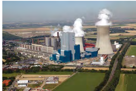
► Power plant in Niederaussem, Germany: A modern lignite-fired 1,000 MW el unit in the foreground and (up to) 40-year-old units in the background.
