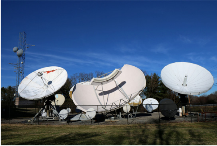
Figure 10.13a Antennas at the studios of the WDBJ television station in Roanoke, Virginia. The reflector antennas are all used for satellite communications. The center antenna is a Simulstat design capable of receiving signals from multiple satellites. The large antenna at the left of the photograph has a Gregorian configuration with a shaped subreflector. The two antennas on the mast link to WDBJ's broadcast antenna on Poor Mountain. For a color version of this figure please see color plate section.
