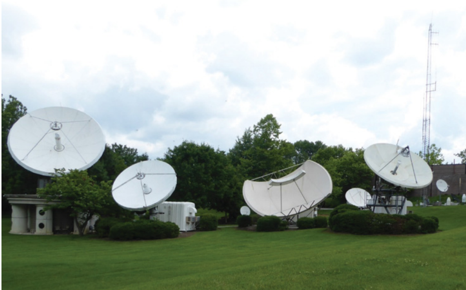
Figure 10.1 Virginia Tech earth station. The two Cassegrain antennas in the left of the photograph are a 9 m C-band steerable antenna and a 5 m Ku-band steerable antenna with dual polarization uplink transmitters. The parabolic torus antenna in the center of the picture is a Simulsat antenna that can receive signals from seven satellites simultaneously. At right is a repositionable Ku-band Cassegrain antenna. Source: Photo credit: Tim Pratt. For a color version of this figure please see color plate section.
