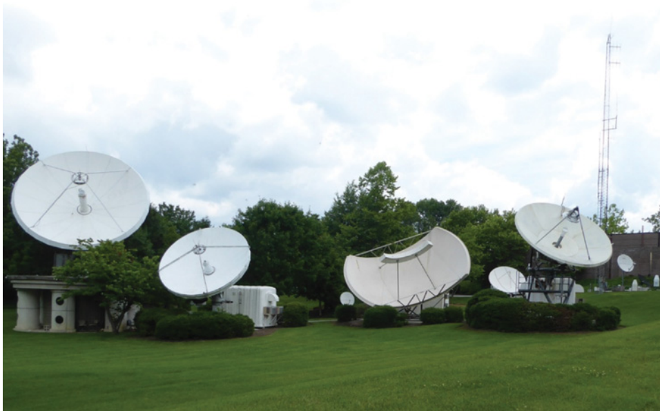
Figure 10.1 Virginia Tech earth station. The two Cassegrain antennas in the left of the photograph are a 9 m C-band steerable antenna and a 5 m Ku-band steerable antenna with dual polarization uplink transmitters. The parabolic torus antenna in the center of the picture is a Simulsat antenna that can receive signals from seven satellites simultaneously. At right is a repositionable Ku-band Cassegrain antenna. Source: Photo credit: Tim Pratt.
