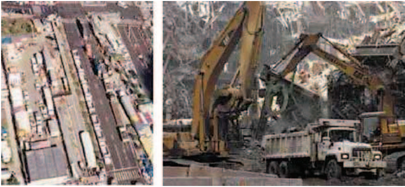
Fig. 3. A typical construction yard scenario.
