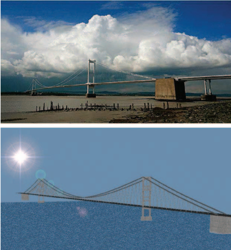
Fig. 2. Photograph and a computer simulation of the Severn Suspension Bridge, UK.
