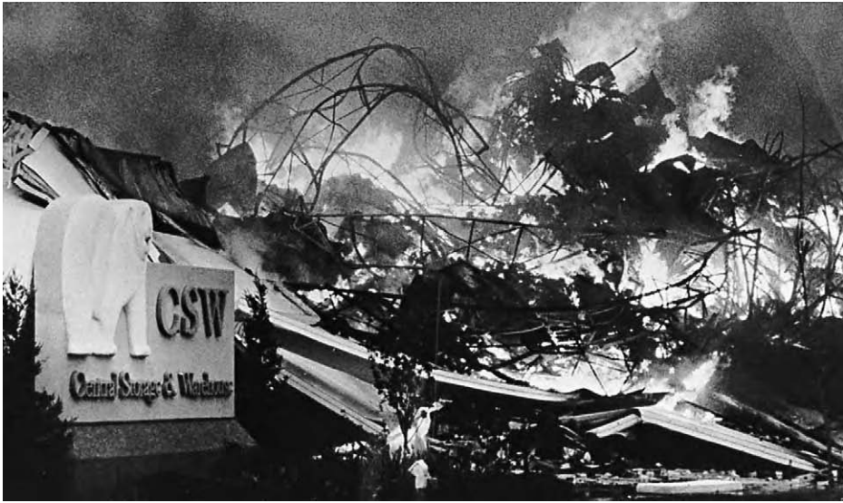
Figure 11-1 A fire in this warehouse in Madison, Wisconsin, caused tens of millions of dollars in damage and kept broadcast news organizations busy for days. (Photo by Kathy Ozatko. Used by permission of the Capital Times )
