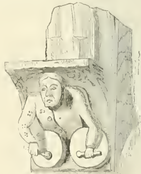
Corbel: Duston, Northamptonshire.
