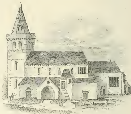
Crail Church (before the restoration).
