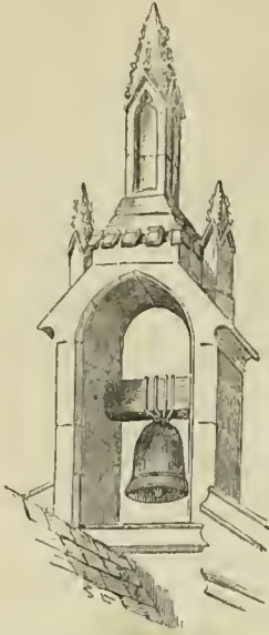
Belfry or Bell-gable, Idbury, Oxfordshire
