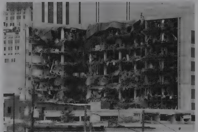
The ruins of the Alfred P. Murrah Federal Building in Oklahoma City
