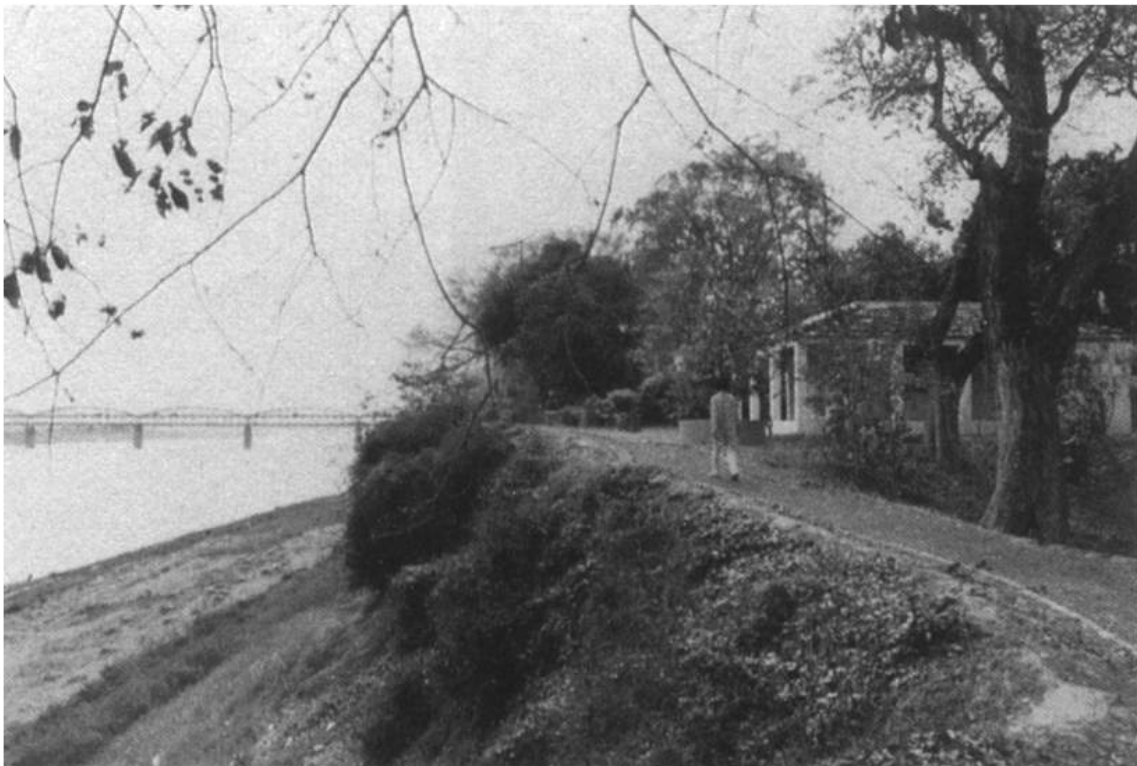
View from K's bedroom at Rajghat
