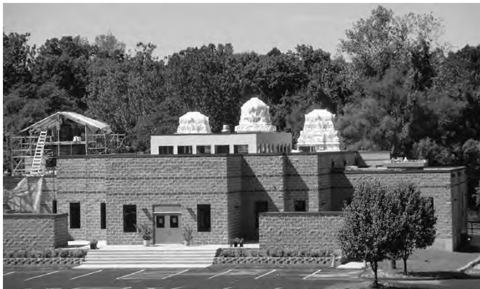
A Hindu temple in progress, St. Louis, Missouri, 1998. A simple concrete block structure begins its transformation toward an elaborately decorated place of worship in Southern temple style, scheduled for completion in 2000. The fourth of five planned spires rises over the inner shrines or “womb chambers” ( garbha griha ) housing the principal deities. Soon the building will have a fifty-foot-high “royal gateway” ( raja gopura ).
