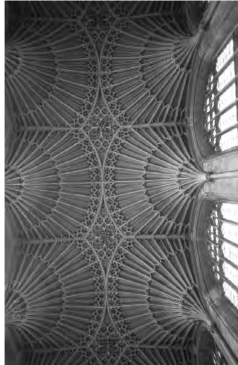
Fan vaulting in the Cathedral of Bath, England, twelfth century; one of many decorative treatments that developed along with advances in the sophistication of engineering for Gothic vaulting.
