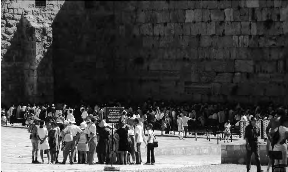
Western Wall of the Jewish Temple, popularly known as the “Wailing Wall” because of its association with annual lamentation on the Ninth of Av over the destruction of the Temple. The lower courses of masonry are from Herod’s time, identifiable as Herodian by the trimmed outer margin of each stone.
