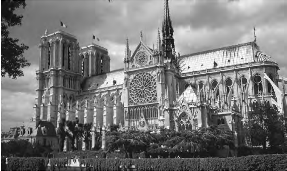
Medieval Gothic style Cathedral of Notre Dame, Paris. The flying buttresses allow extensive wall space for stained glass, and the huge mandala-like “rose window” over the south transept is rich with Biblical symbolism.
