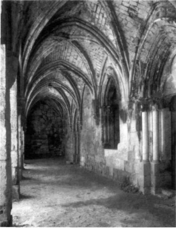
Crac: interior of the loggia.
