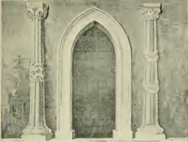
COLUMNS AT WÜRZBURG CATHEDRAL, BAVARIA.
