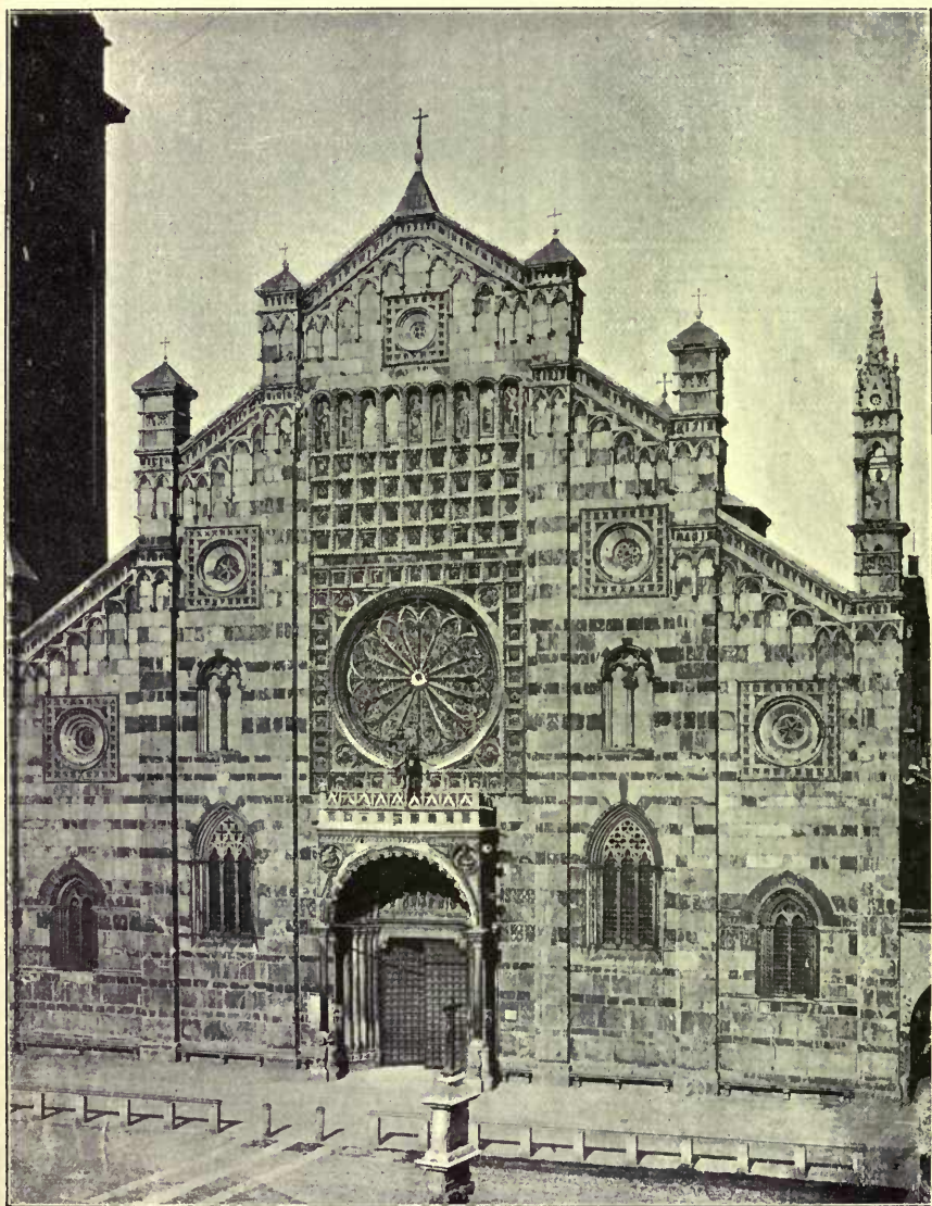
FAÇADE OF MONZA CATHEDRAL. RESTORED 14TH CENTURY.
