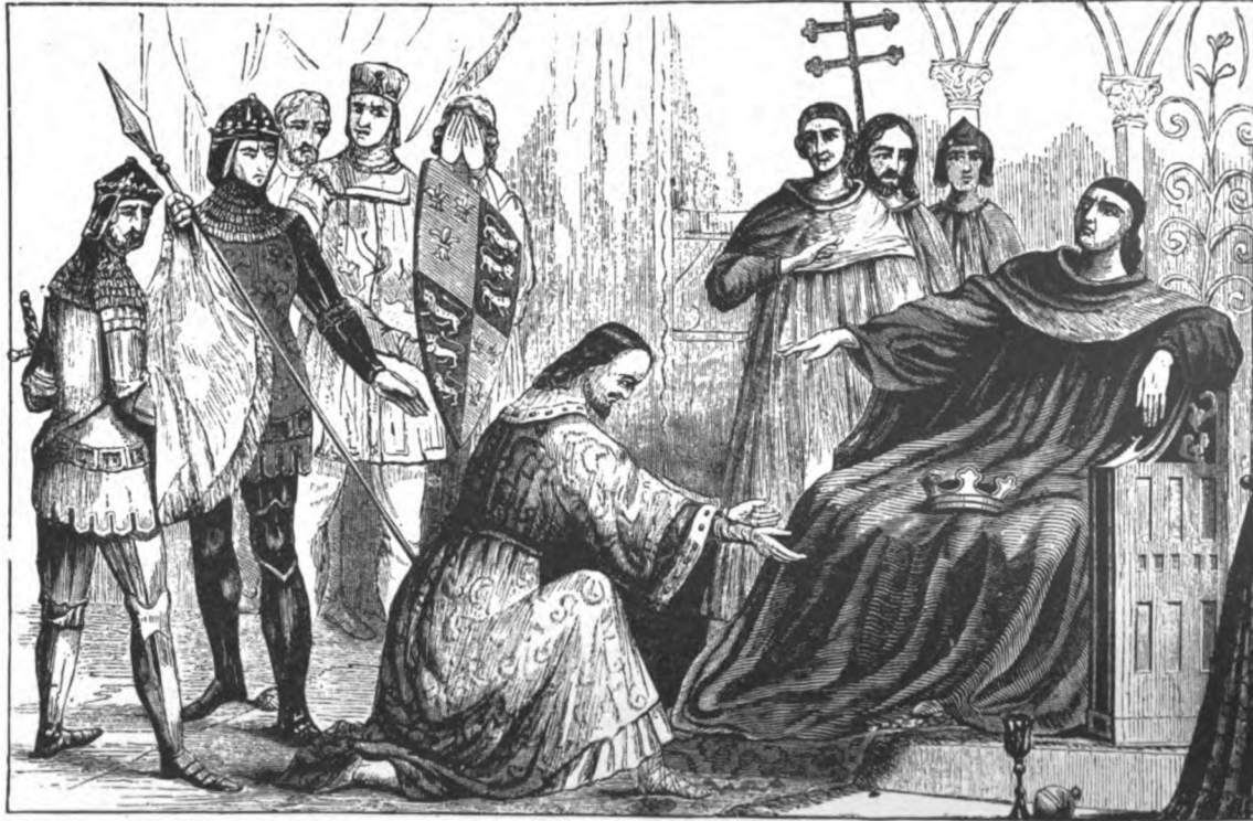
King John degrading himself.
