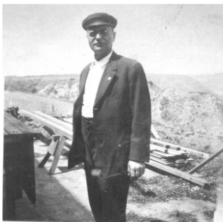
64. Mr Heindel during the building activities in 1913.
