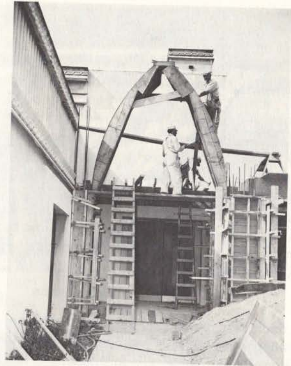
The Judkins brothers at work on the Mayan style arch over the entrance of the PRS Library.
