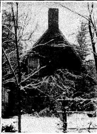
Below: Front of the Tappan Shrine, showing, left, a frame structure erected subsequent to the Revolution. The window in the roof to left of the tree opens from the room which was occupied by Washington.
