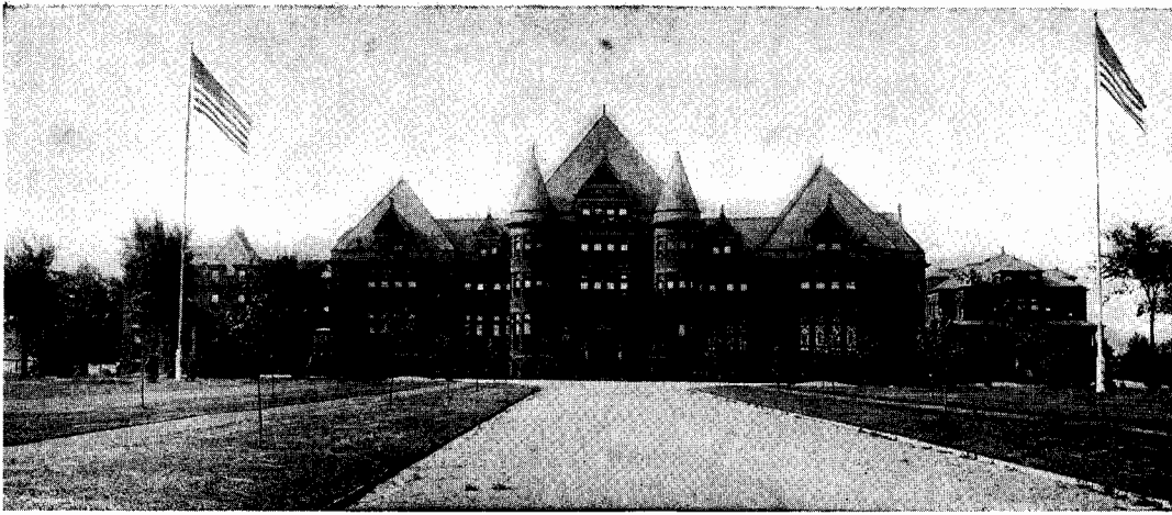
Masonic Home, Utica, New York—The Administration Building.
