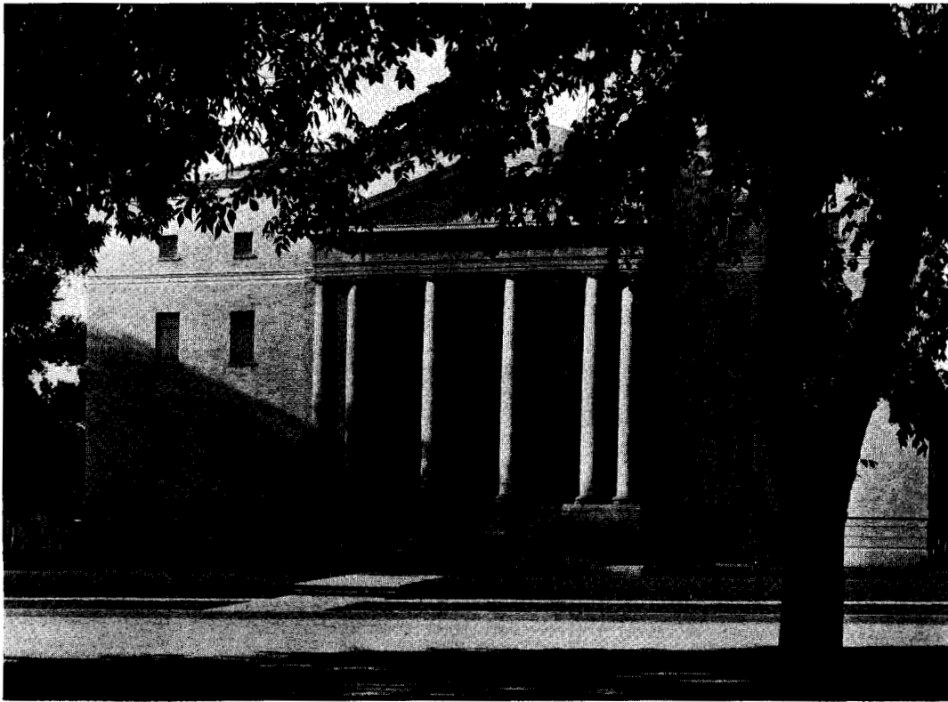
Masonic Temple, Fort Collins, Colorado.
