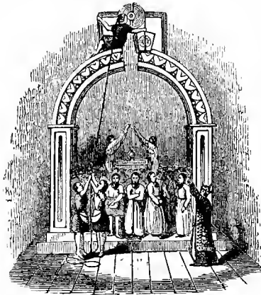
PLACING THE KEYSTONE.
