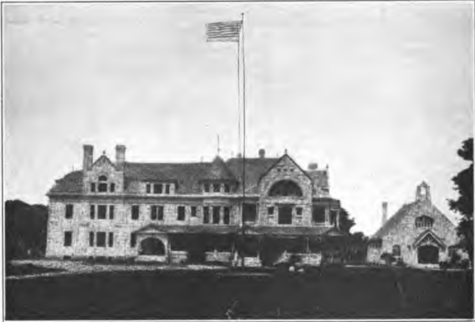
KANSAS MASONIC HOME RECENTLY DESTROYED BY FIRE
