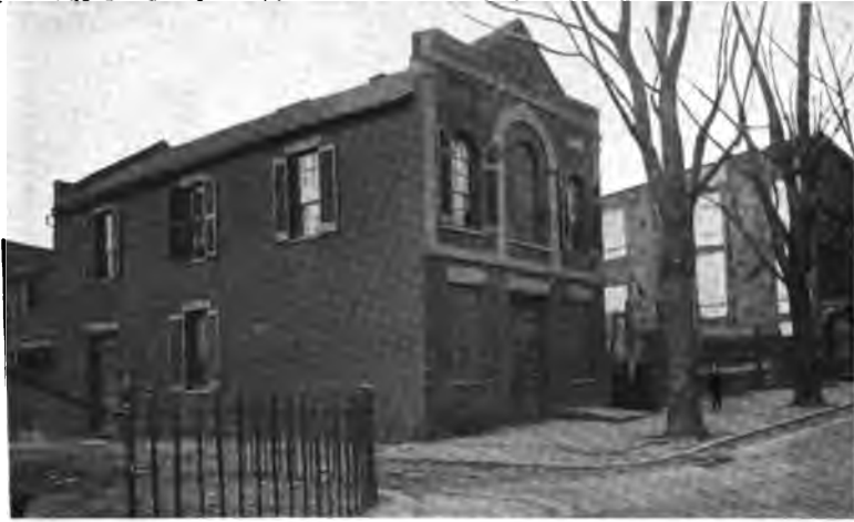
MASONIC HALL, JEFFERSON STREET, GEORGETOWN, D. C. Home of Potomac Lodge, No. 5, 1810 to 1840.
