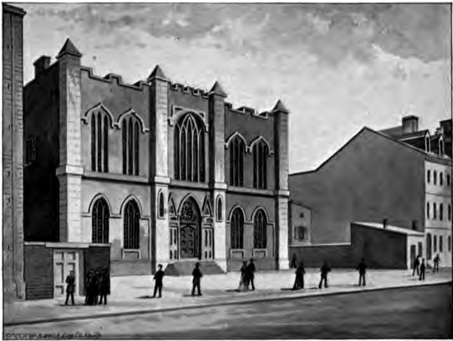
The Second Hall on Chestnut Street, 1820-1835.
