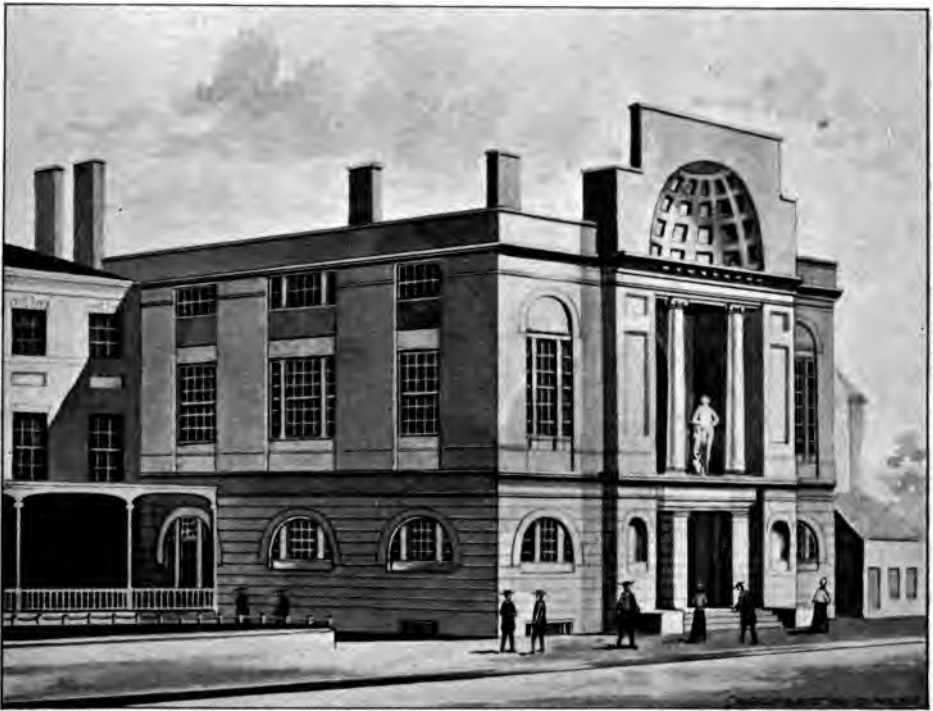
The Hall on Third Street. 1835-1855.
