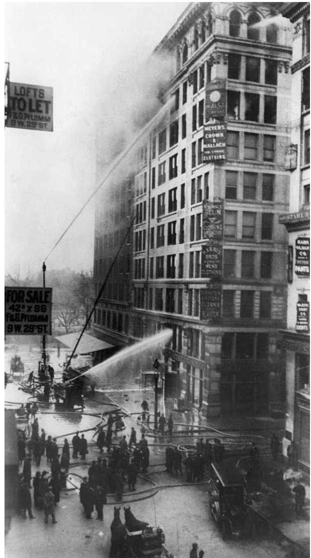
The high death toll of the Triangle Shirtwaist Company fire was a result of locked doors and inadequate fire escapes. New federal safety regulations were established to reduce the likelihood of other such disasters. UNDERWOOD & UNDERWOOD/CORBIS
