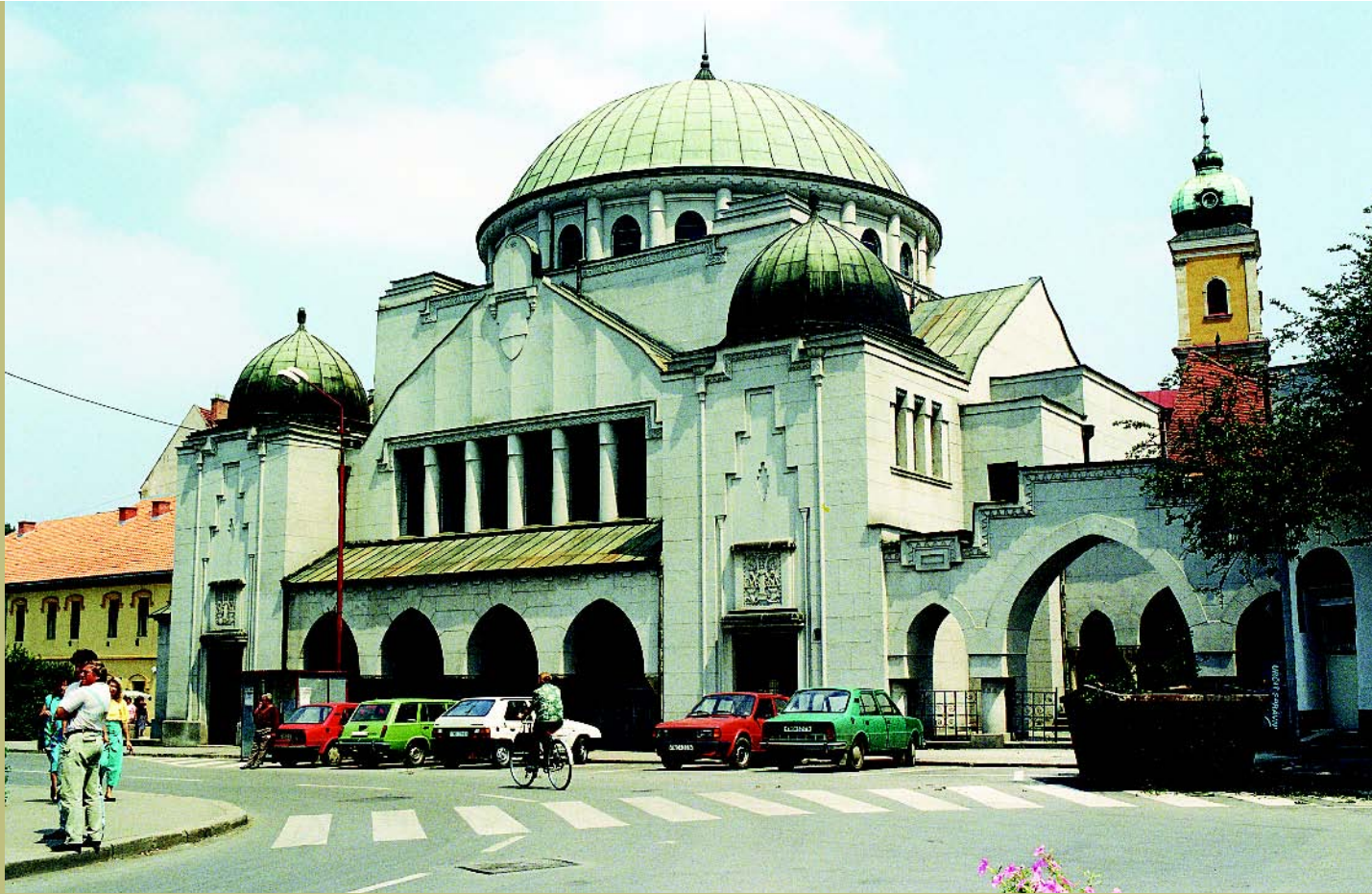
Synagogue (now an art gallery) in Trencin, Slovakia. This imposing edifice was completed in 1913 to replace a 125-year-old building and to serve the needs of some 1,500 Jews, about 16 percent of the town's population. With lavish dome and Oriental decorative motifs, the synagogue contains a spacious winter prayer-room on the southern side, shown here, where a small kehillah of fewer than two dozen members met weekly for Shabbat prayers in the 1990s. Photo: Rivka and Ben-Zion Dorfman, Synagogue Art Research, Jerusalem.
