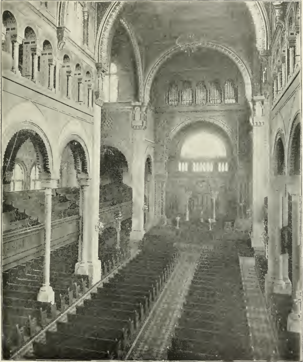
INTERIOR OF TEMPLE EMANU-EL, FIFTH AVENUE, NEW YORK. (From a photograph.)
