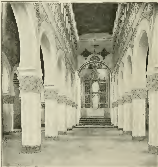
Interior of the Church of St. Maria la Blanca, Toledo, Formerly a Synagogue. (From a photograph.)
