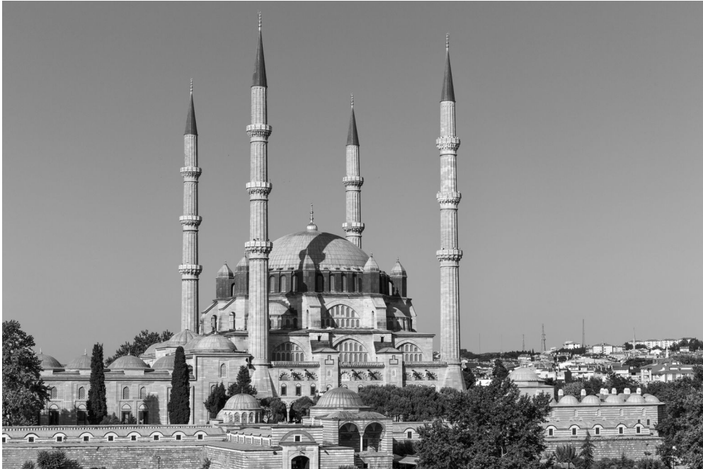
The Selimiye mosque in Edirne, Turkey was the great architect Sinan's last major work. While its dome is wider, the building stands forty feet shorter than the Hagia Sophia.
