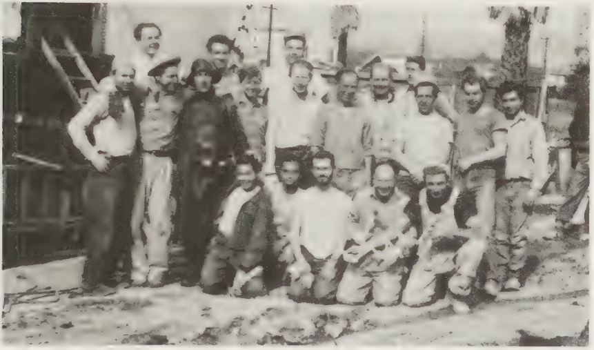
The monks working on building India Center in 1951.
