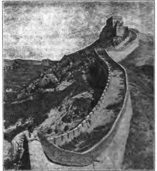
LOOKING EAST ALONG THE GREAT WALL
