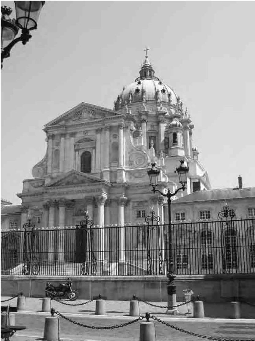
Figure 3 Val-de-Grace, Paris. The church was built between 1645 and 1667. The work was commenced by the architect François Mansart and completed by Jacques Le Mercier. The cupola was designed by Pierre Mignard. (Photograph by Helen Chenut.)
