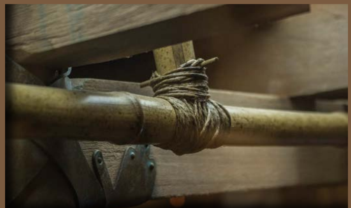
Liquid waste would move into the bamboo piping and away from the enclosures
